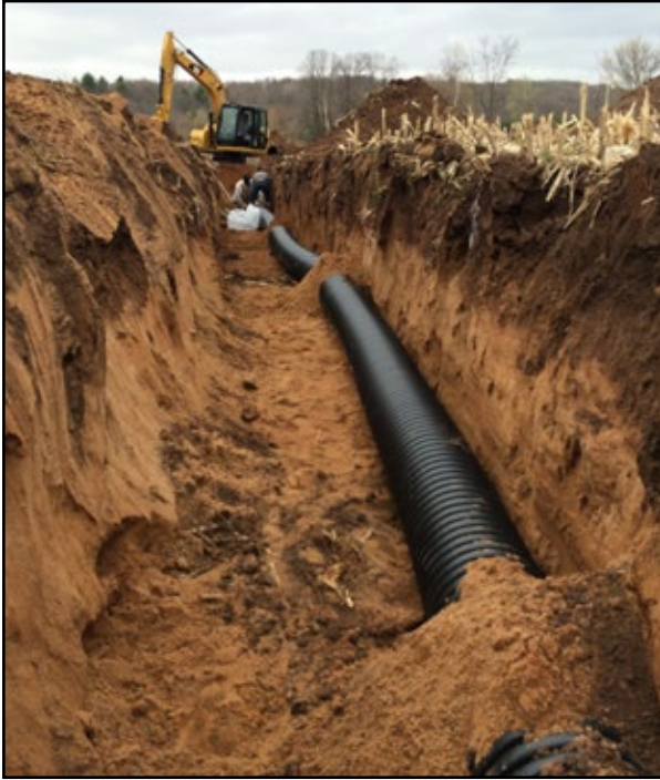
Installation of water and sediment control basin
