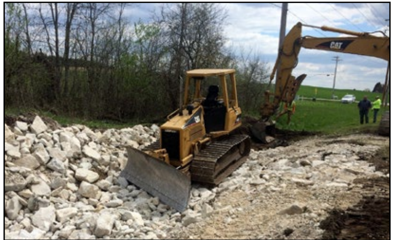
Installation of a large lined waterway in Sheboygan County
