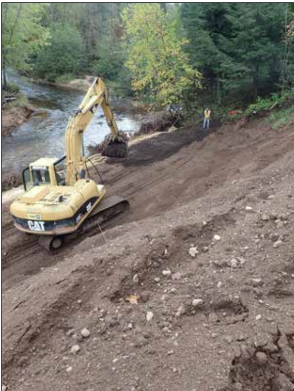
Bluff restoration in Bayfield County that required moving the river over 30 feet and installing hundreds of log deflectors. Project completed by Bayfield County in partnership with Northland College, U.S. Fish and Wildlife Service, Town of Lincoln, WI DNR and the Superior Rivers Watershed Association. Photo: Bayfield County
