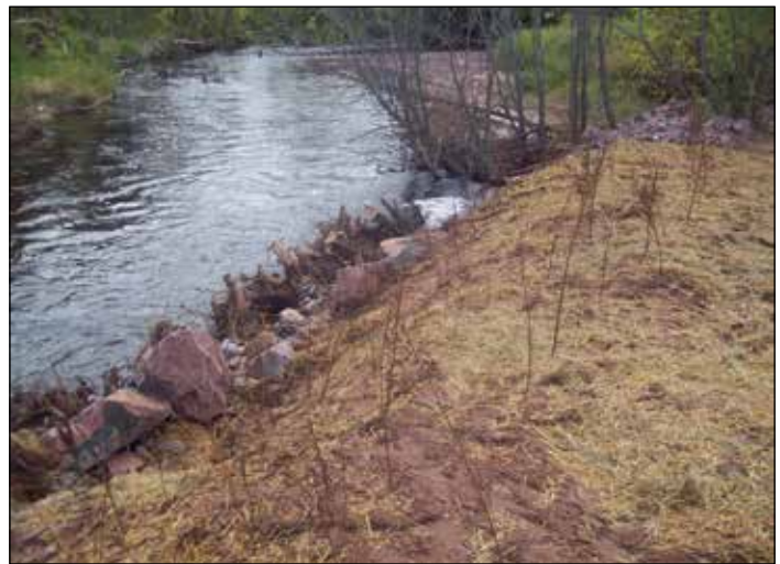
Root wads installed as part of an erosion control project on the Brunsweller River in Ashland County. The project reduces sedimentation concerns and improves aquatic and terrestrial habitat. Funding for the project from WI DNR, NRCS, and DATCP. Photo: Ashland County
