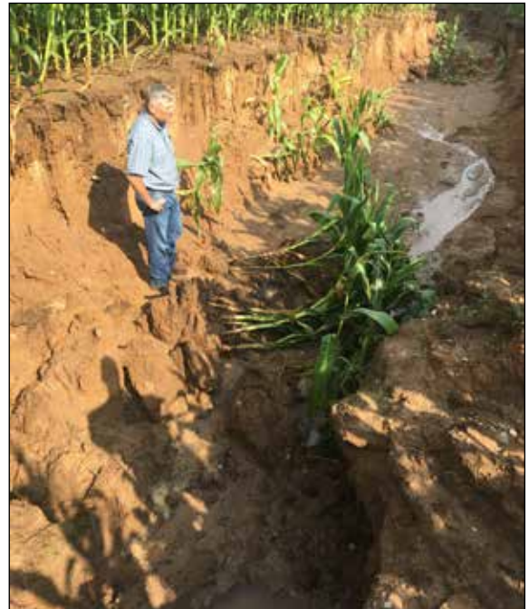
A single rainstorm that dropped 7 inches in a few hours scoured this gully and two others out of a slope planted to corn. Photo: Oconto County Land Conservation Department
