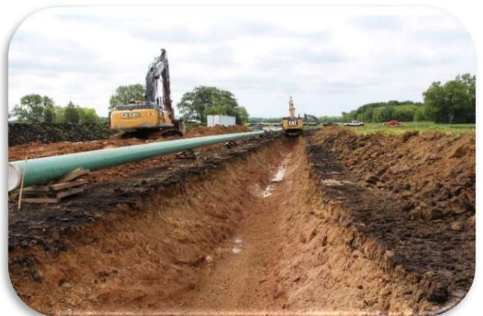
Figure 6: Open trench excavation.
