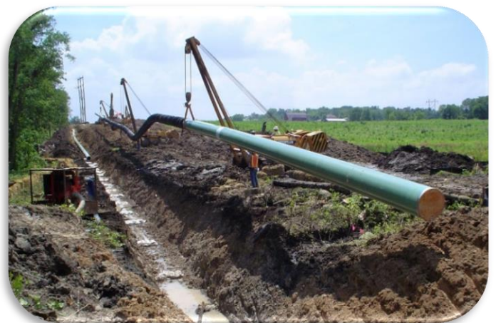
Figure 7: Lowering of pipe into open trench.
