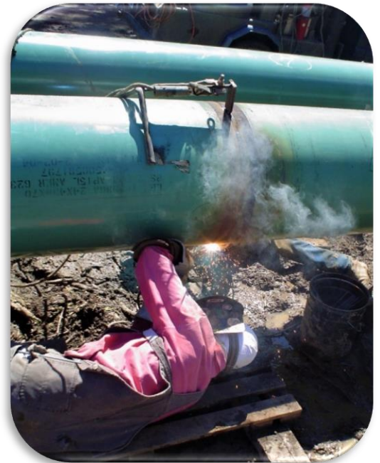
Figure 5: Pipe welding within the ROW.
