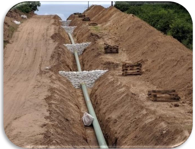
Figure 8: Placement of sandbag trench breakers.
