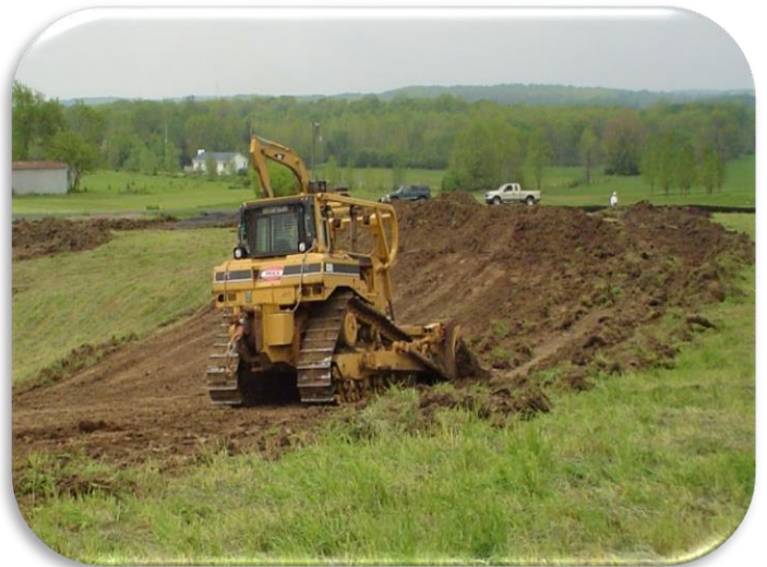
Figure 3: Topsoil stripping.
