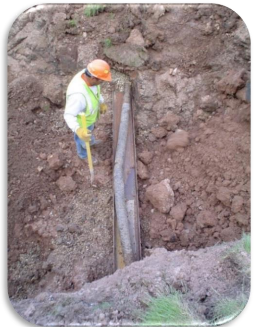
Figure 9: Drain tile repair made with flexible drain pipe and steel channel.
