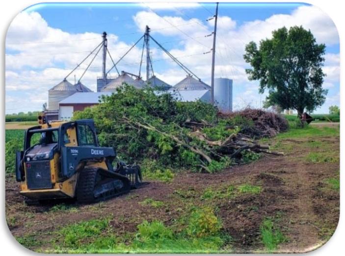
Figure 2: Removal of trees and shrubs from ROW.
