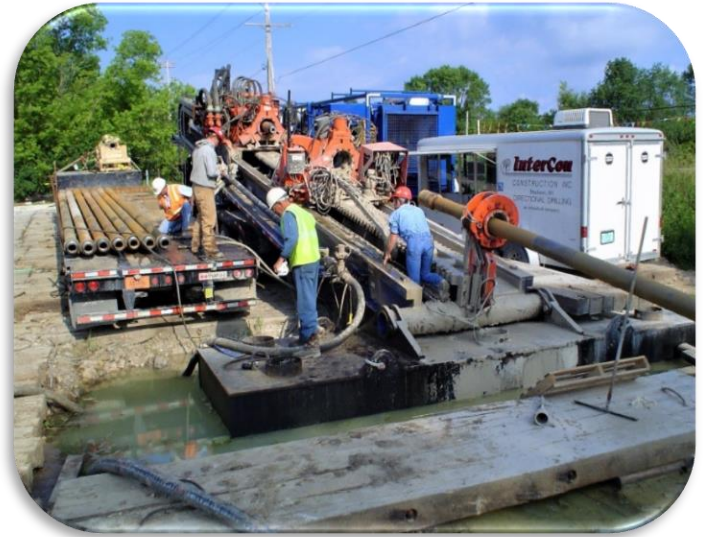
Figure 10: A horizontal directional drill machine.
