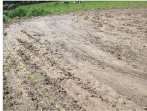
Poor infiltration, deposition
